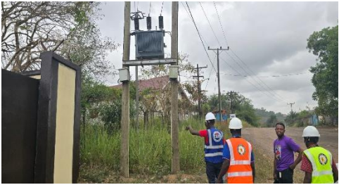
Rectified Leaning Transformer
