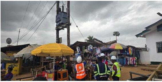
Marketers Under Transformer in Gbali
